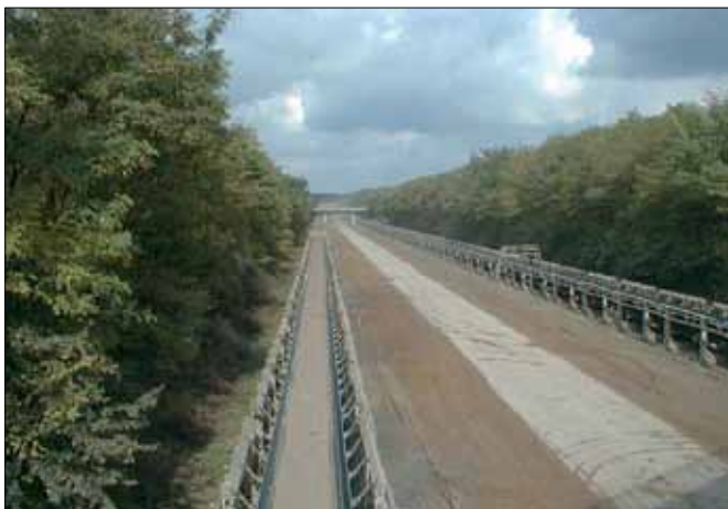
Fig. 3: Overburden transport from Hambach to Bergheim via long-distance conveyor belt
